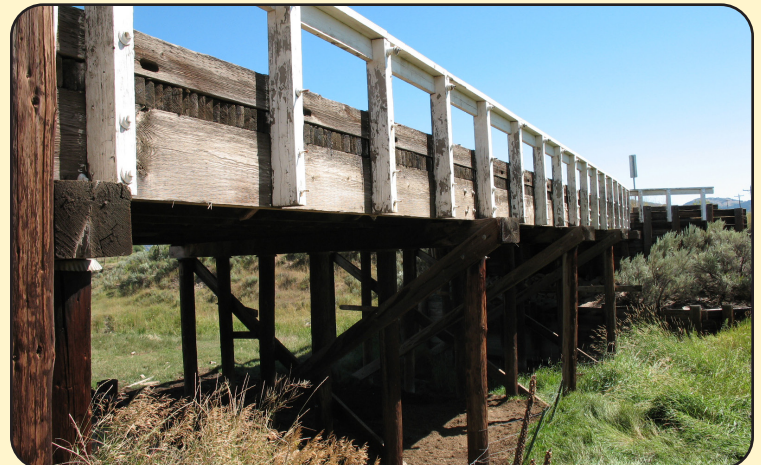
Image 8. SH 64 over Strawberry Creek in Rio Blanco County
