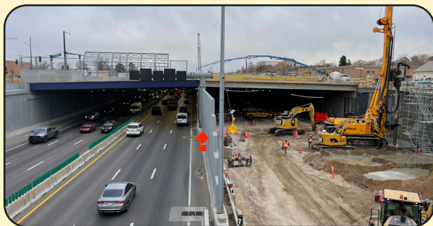
Image 26. Construction of the Lowered Eastbound I-70 Lanes
