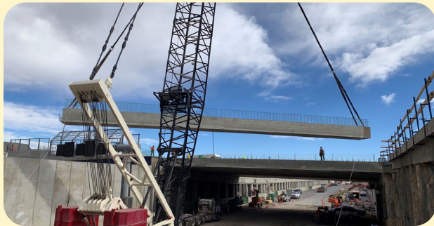
Image 25. Setting the Girders for the Lowered Eastbound I-70 Lanes
