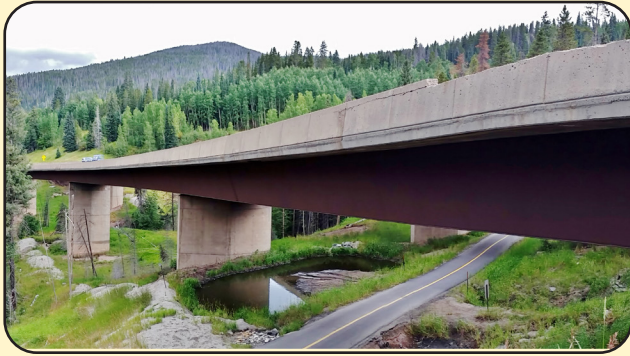
Image 30. I-70 EB over Polk Creek in Eagle County (F-12-AS)
