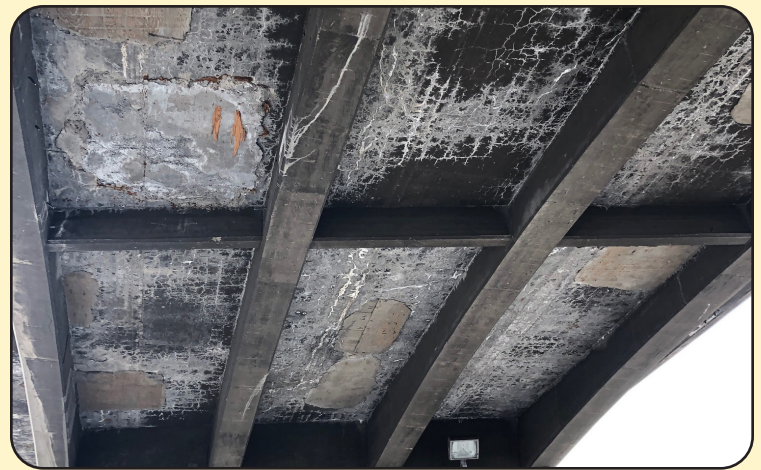
Image 3 & 4. Deteriorated Concrete on I-76 over York Street in Adams County
